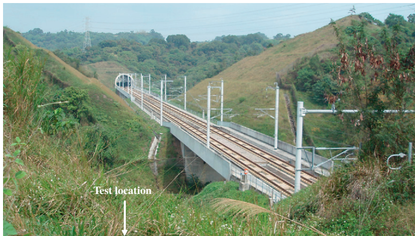
Fig. 11. Location of the experiment near a complicated site with an embankment, a bridge, and a tunnel.
