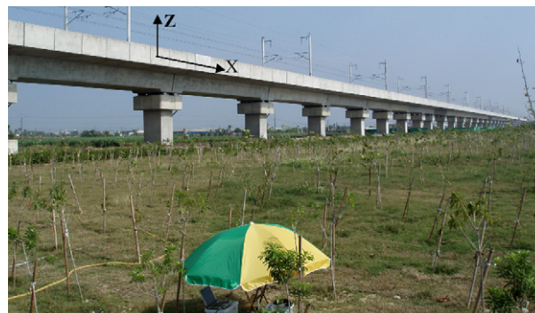
Fig. 6. Field experiments for measuring train-induced vibrations on simply supported bridges.
